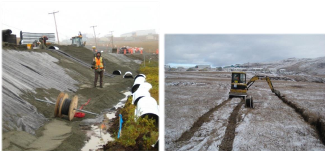
Figure 6 : Installation of the fiber optic cable in 2012 (Lemieux et al., 2013)
