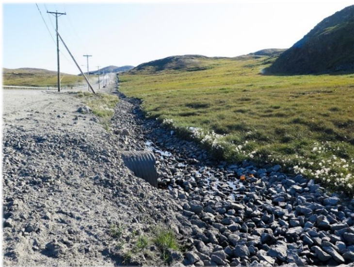
Figure 5 : The gentle slope technique and the interceptor ditch protected by riprap implemented on the road west side (August 2017).
