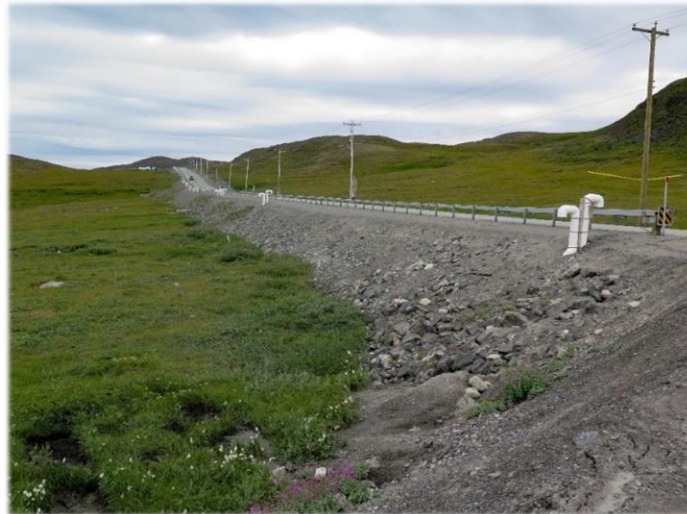
Figure 3 : Heat drain mitigation technique, east side of the road (August 2017).
