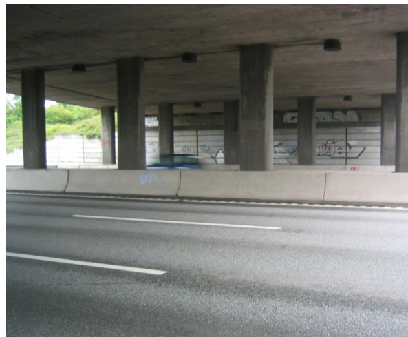
Concrete safety barrier
