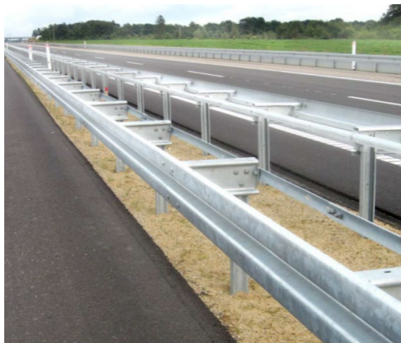
Steel safety barrier
