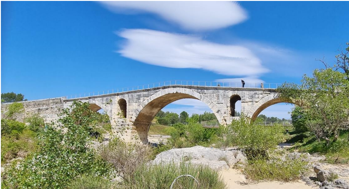
Figure 4-6: Pont Julien – Via Domitia – France – year 3 BC - Span 46 m
