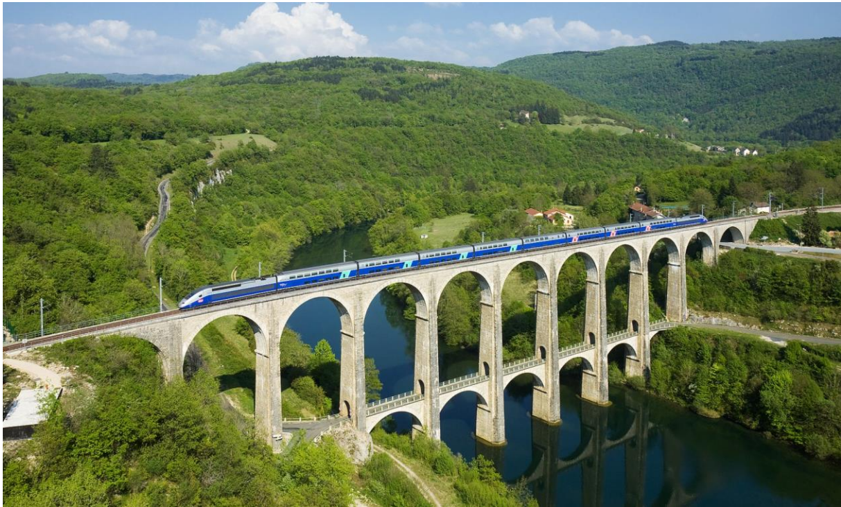
Figure 1-1: Viaduc de Cize-Bolozon - France
