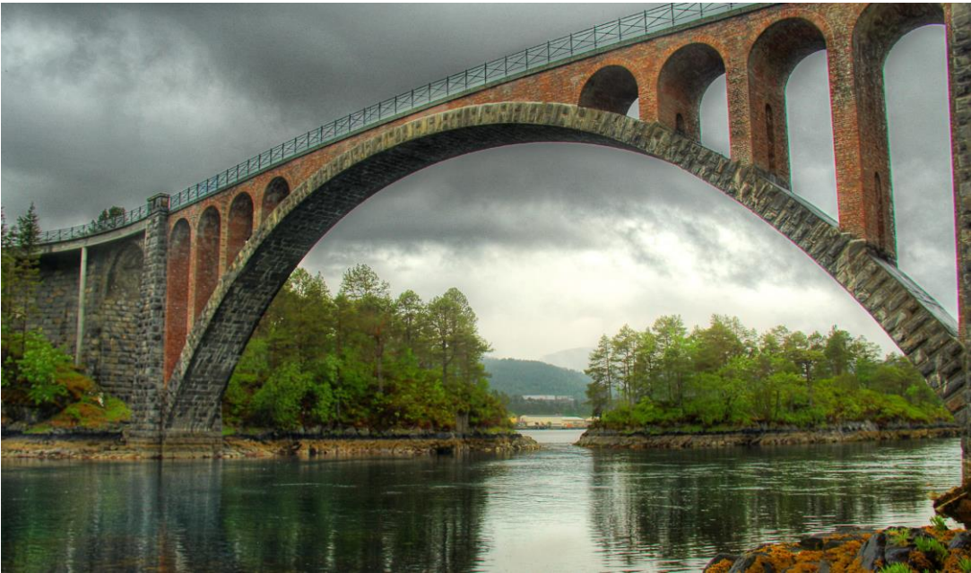
Figure 3-1: Skodje bridge - Norway – 1922 - arch span 57 m
