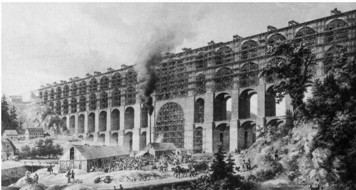
Figure 2-10: The Göltzsch viaduct in Germany - 1851
