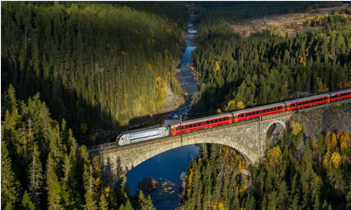
Figure 2-12: Orkla railway bridge - 1916
