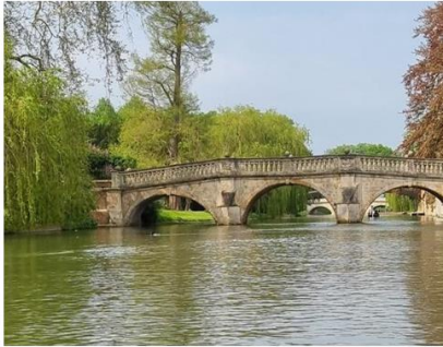
Stone arch bridge, Cambridge
