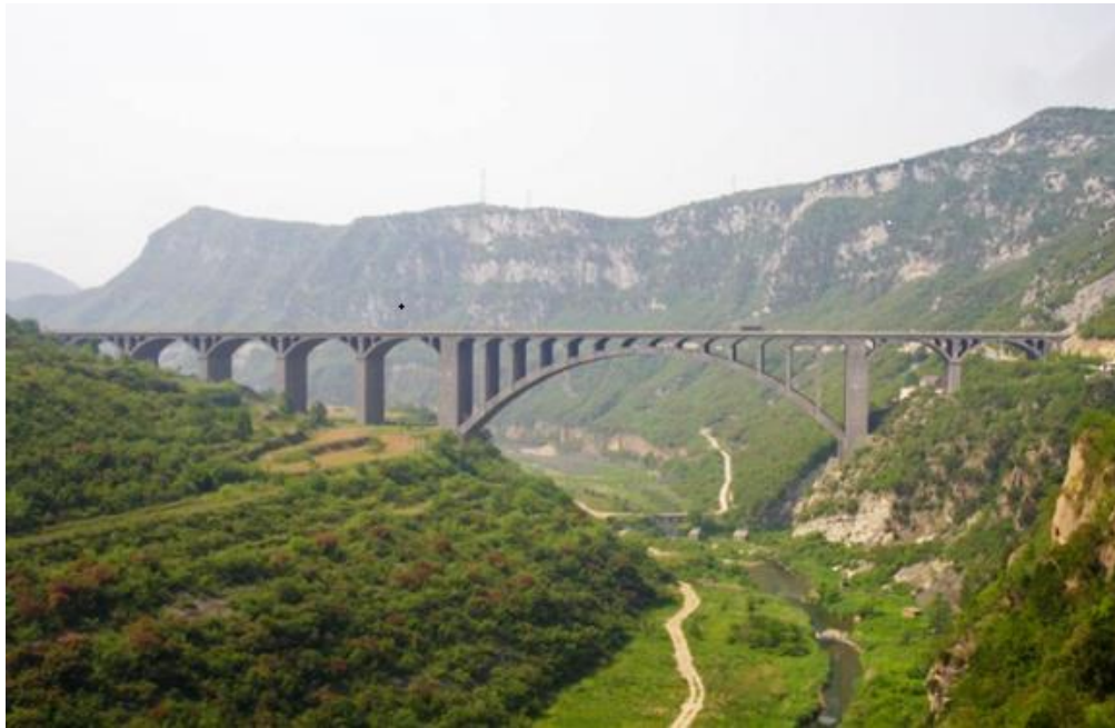
Figure 3-5: Dahne bridge - China
