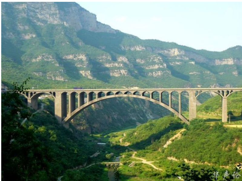
Figure 2-15: Dahne bridge – 4 lane motorway – 2001 - China
