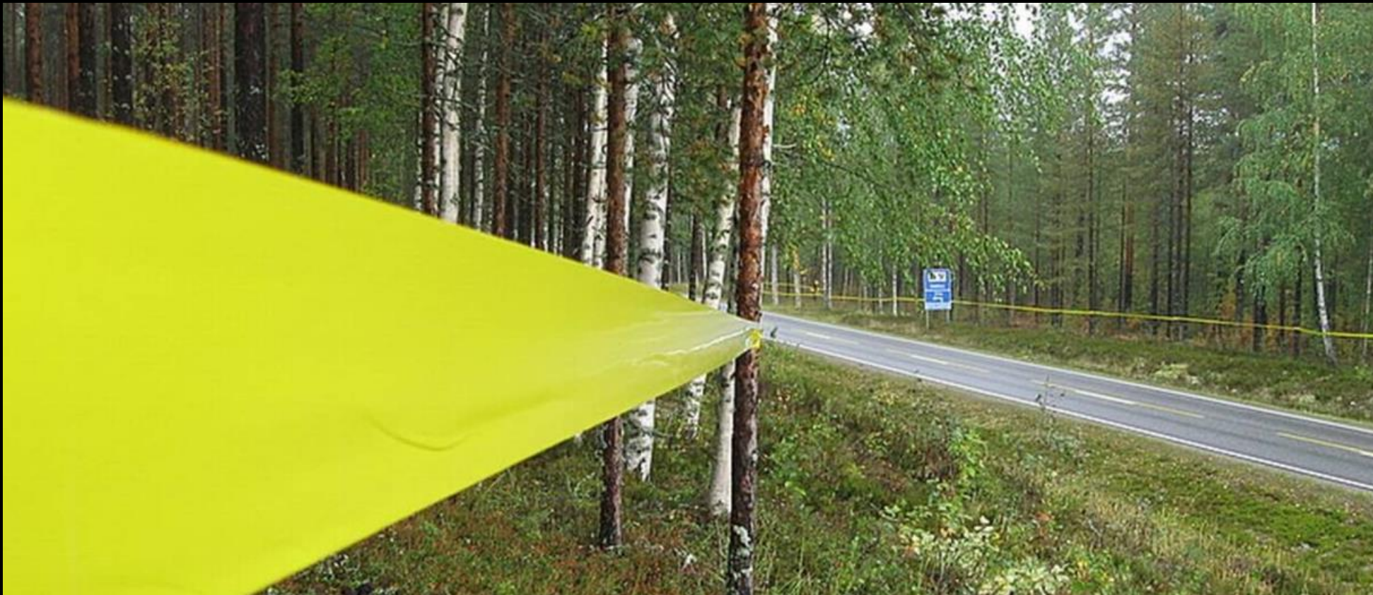
Figure 11 - Moose and deer tape should be placed in a highly visible position at the roadside so that the moose or deer can see the tape well before the roadside.
