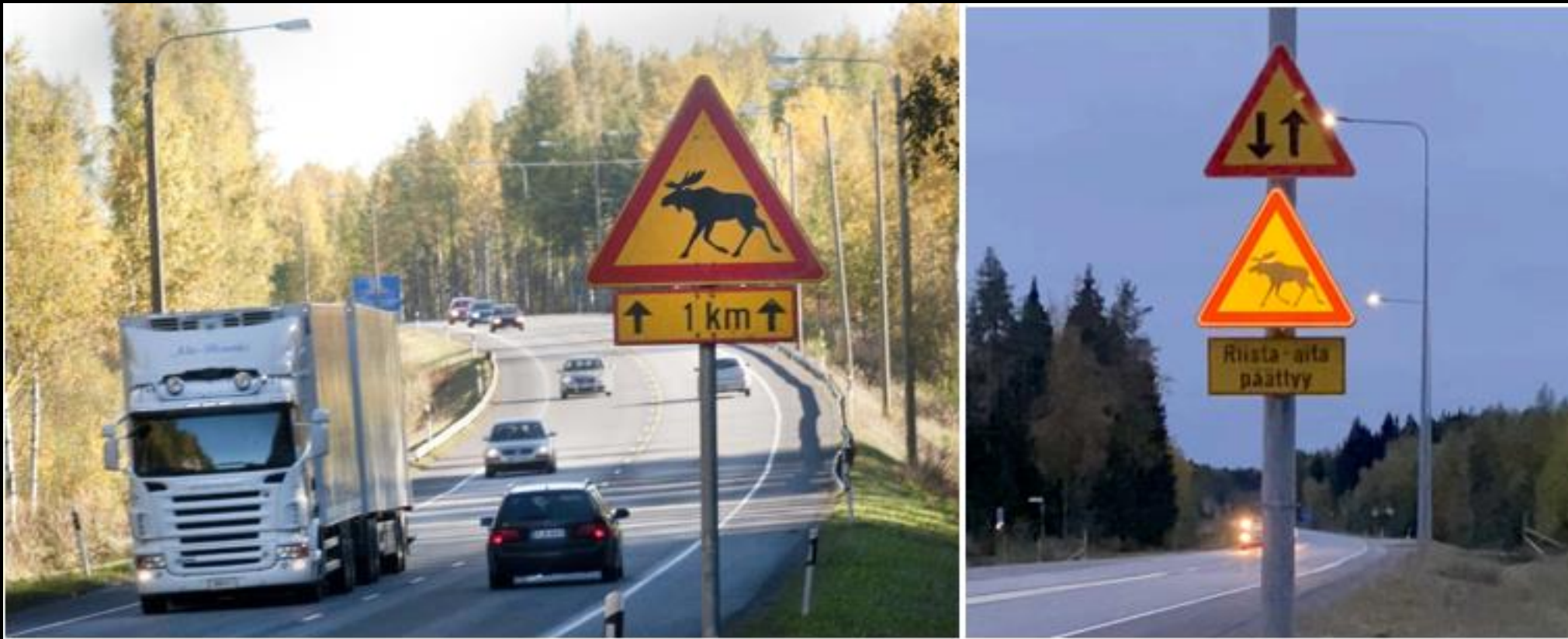
Figure 6 - Passive Road signs always have a fixed message, although they may use beacons or other enhancement devices.
