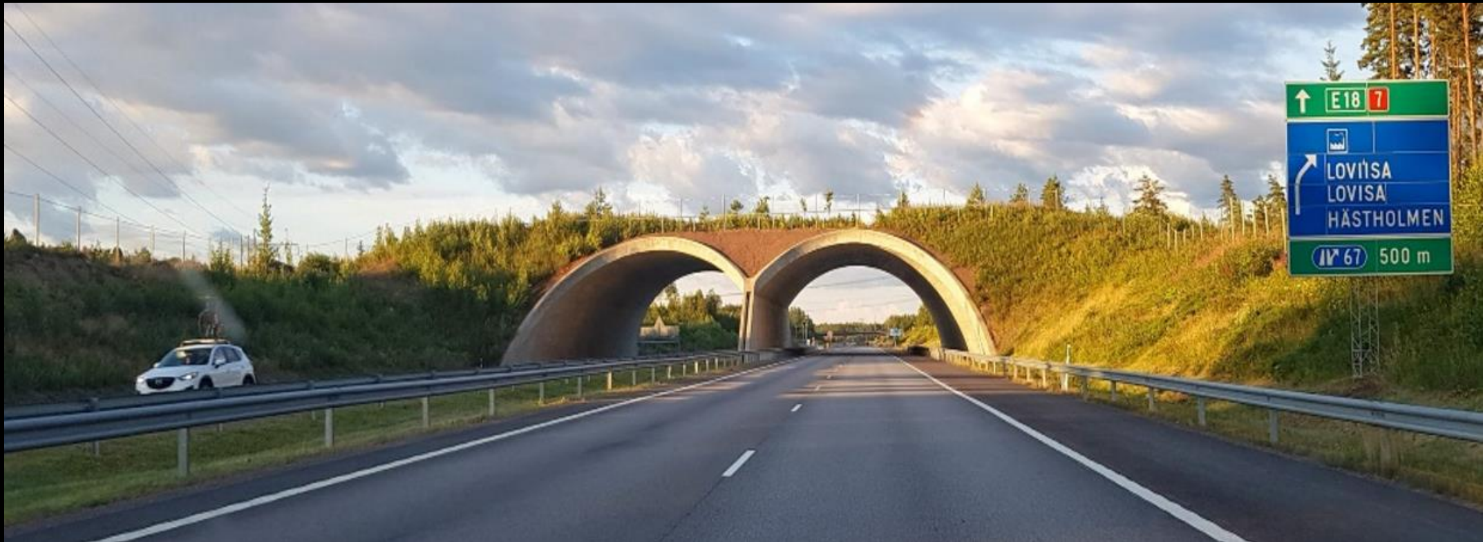
Figure 12 - Green bridges and other animal access structures provide a safe route for animals to cross the road.
