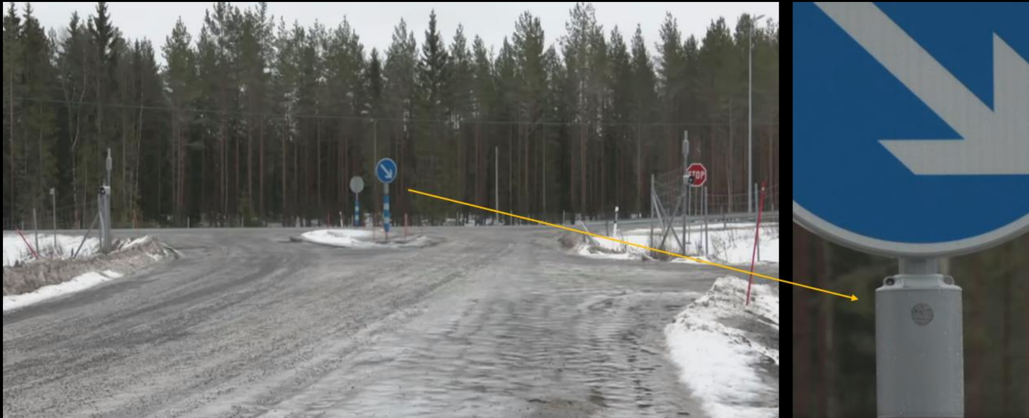
Figure 15 - The loudspeakers at the Vassori level crossing on Highway 8 play a human voice when sensors detect an approaching deer. The goal is for the sound to scare the animal away from the road and back into the forest.
