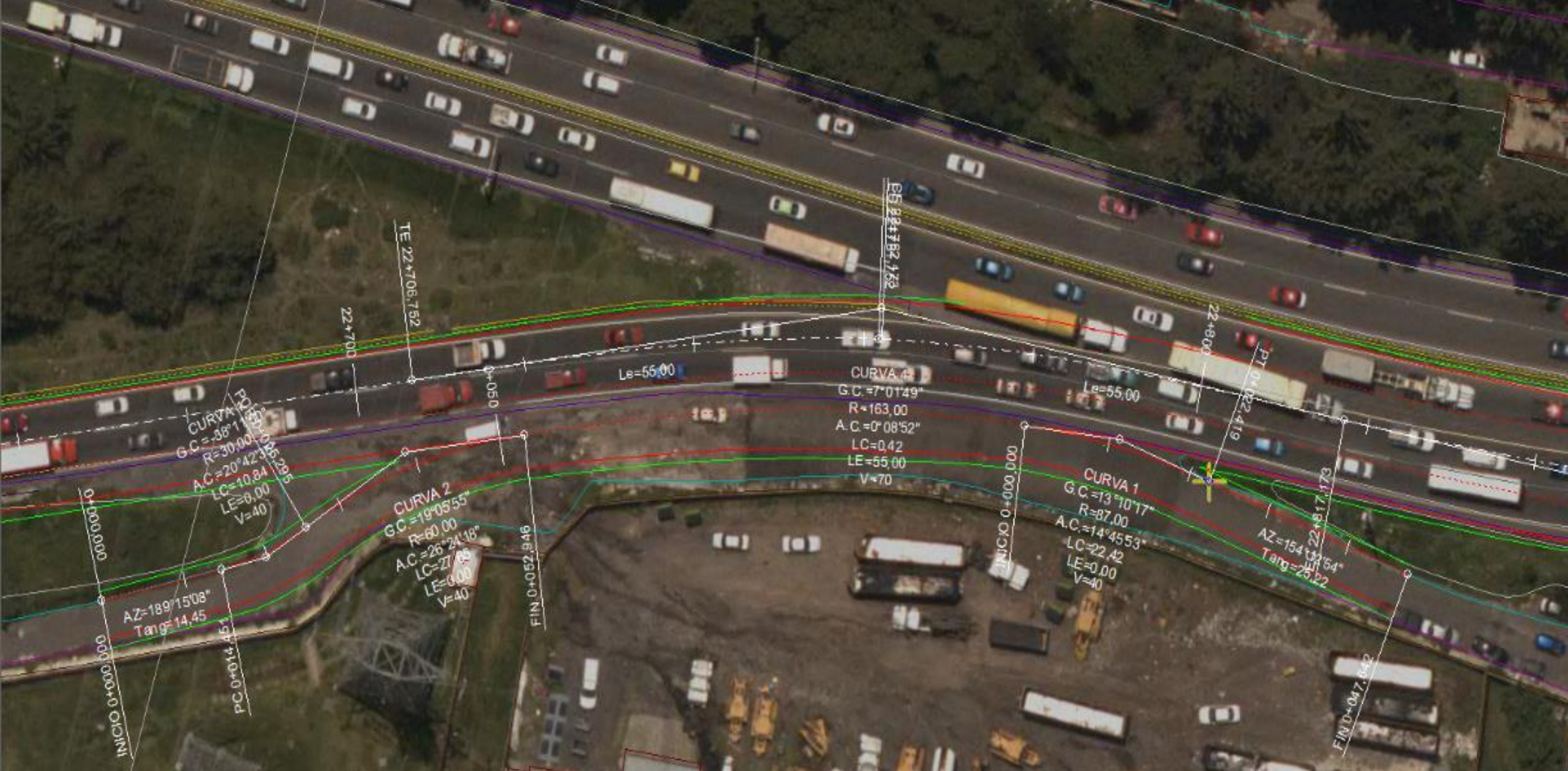
Figure - Connectivity problems with the toll motorway. Road Safety Inspection of the Free Federal Highway Mexico-Toluca (MEX-15), Mexico
