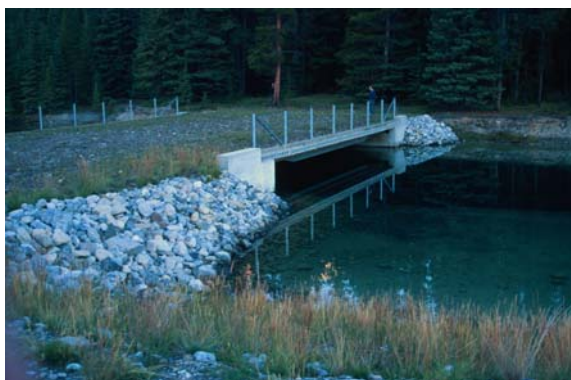
Fig. 21: Viltovergang over vannkanal. Cascade Valley.
