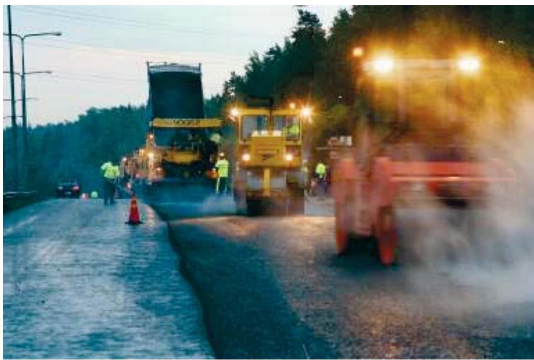
**Fig.2.** Working during the normal laying of SMA from field exposure survey in 1999 /2/.
