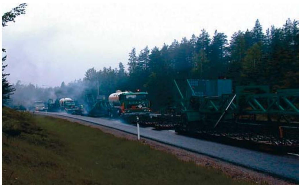
**Fig.3.** Renewing of SMA by the REM-techniques with liquid gas IR-heating system from field exposure survey in summer 2000 /3/
